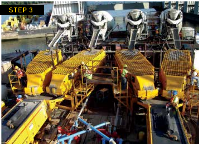
The delivery barges then go to the placing barge where the mixer drums dump the concrete into Maxcrete remix hoppers. The remix hoppers then place the concrete into the hoppers of the BSA 2112 skid-mounted trailer pumps.
