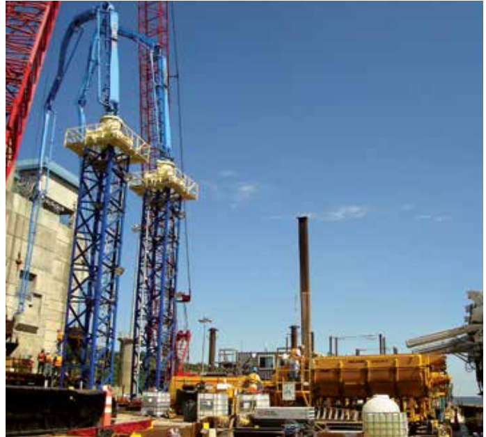
SAB proposed a complete system approach made up of placing booms, truck-mounted concrete boom pumps, diversion valves, remix hoppers and trailer pumps as a solution for placing the tremie concrete.
