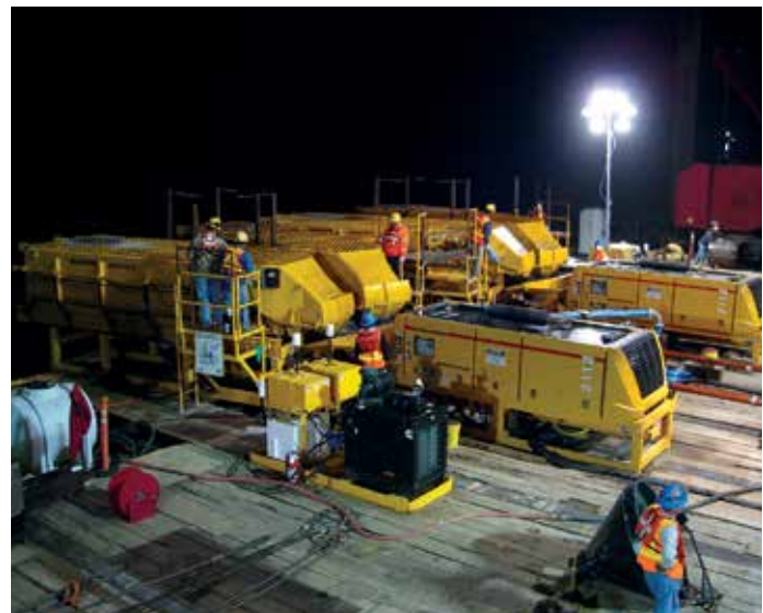
The placement of the concrete for each of the 28 shells is a non-stop 36-hour process.
