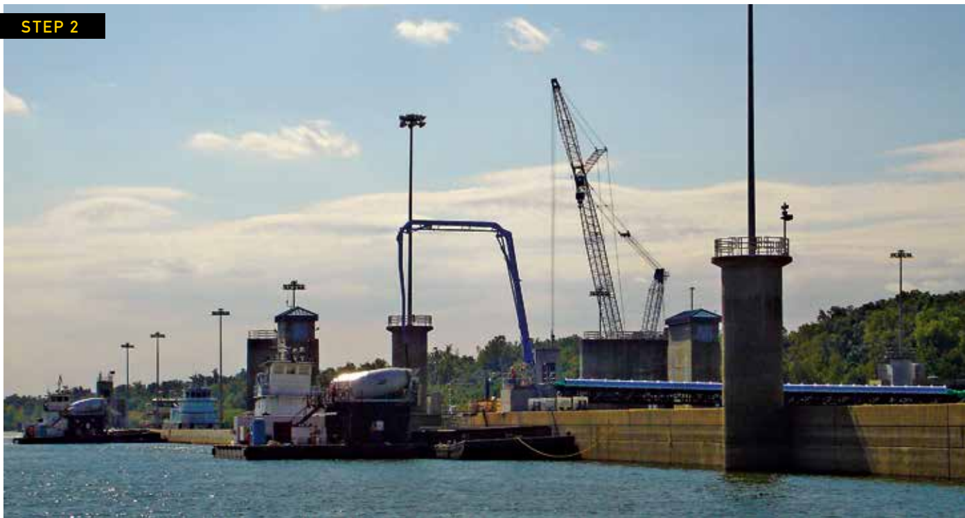
At the end of the slickline is a 312-Meter placing boom, which places the concrete into four stationary mixer drums on each of the two delivery barges.
