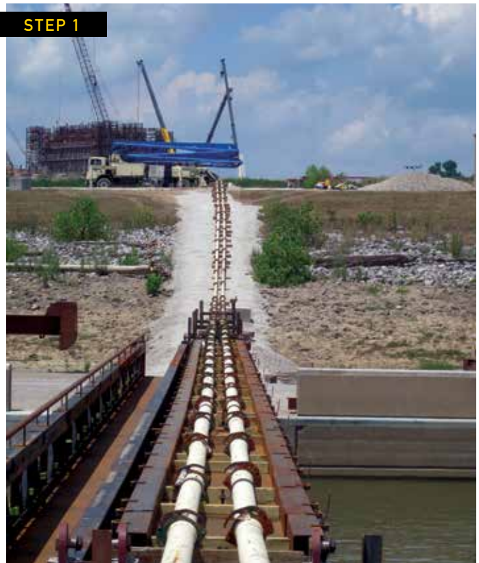
The process of placing the tremie concrete begins with a 40Z-Meter boom pump that delivers the concrete from the river side through slickline across the lock chambers.
