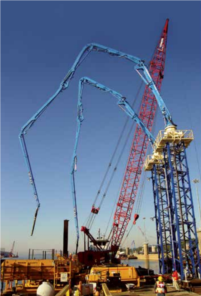
A Putzmeister concrete placing system is placing tremie concrete via the in-the-wet method, a first in the U.S.
