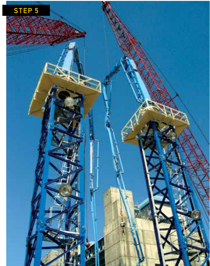
Concrete travels up to the two MX 43/47Z-Meter placing booms where it is placed into the tremie pipes that travel underwater to the concrete's final resting place underneath the precast concrete shells.
