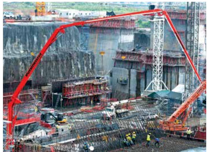
The boom pumps are being used to place a special marine mix.
