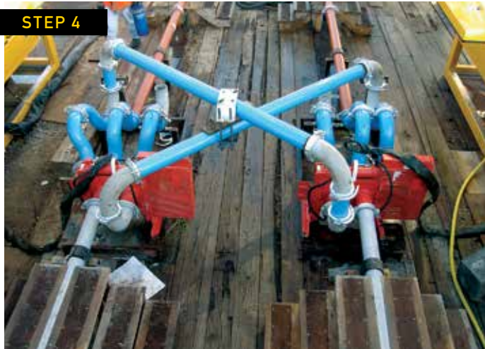
Two DVH 5/2 diversion valves route the concrete pumped by the BSA trailer pumps.
